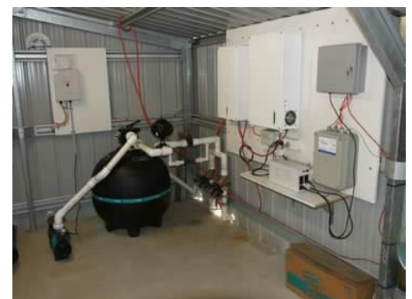
Scotts Tubes NSW, Bottom L to R: propagation house, seed sowing herbs, pump house with ozone water treatment unit
